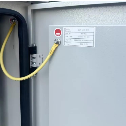
Photovoltaic Power Supply System for
