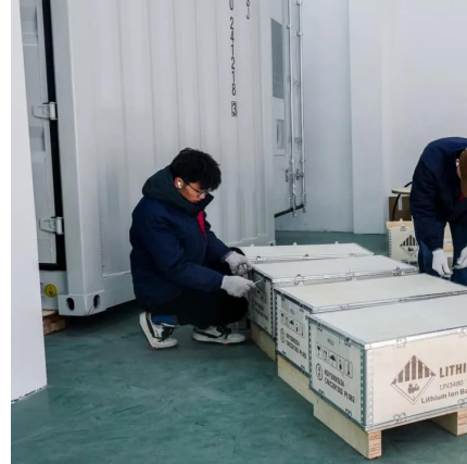
UPS and Battery Bank in Mali , Sempra Electric Pvt Ltd.
