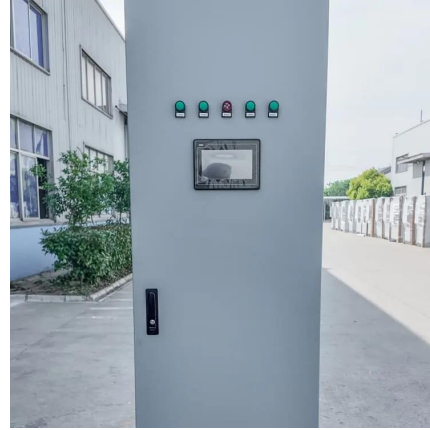
Tesla to build grid-side energy storage station in Shanghai
