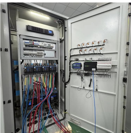
ENERGY STORAGE CHARGING PILE INSTALLATION IN KUWAIT CITY
