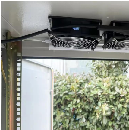
215kWh BESS for Belgian Industrial Factory ...
