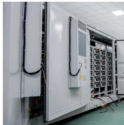
Energy storage system of communication base station
